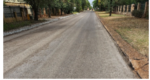
Figure 9(c) Bodenstein Street completed with new slurry seal
