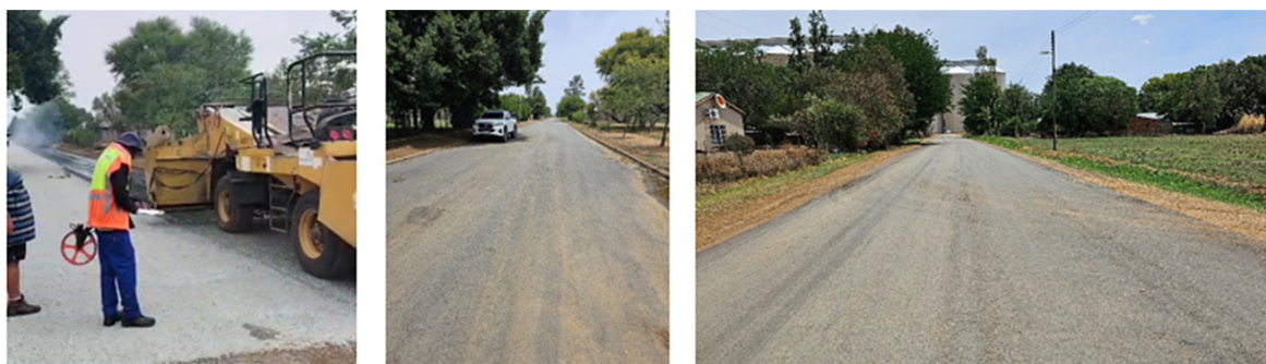
Figure 8: Botha street in Leeudoringstad chip spreading and final surface with slurry show good surface on Botha as well as for West street (link to silos)
