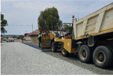
Figure 9(a) Borman street chip and spray operation
