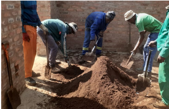
Figure 10: Hand mixing of NME and water
