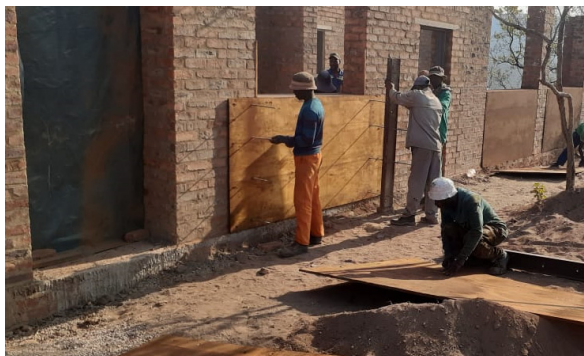
Figure 11: Formwork setup using brick work as solid reference
