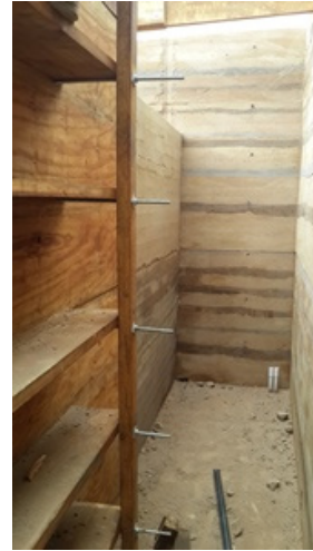
Figure 5: Colour stratification during construction.
