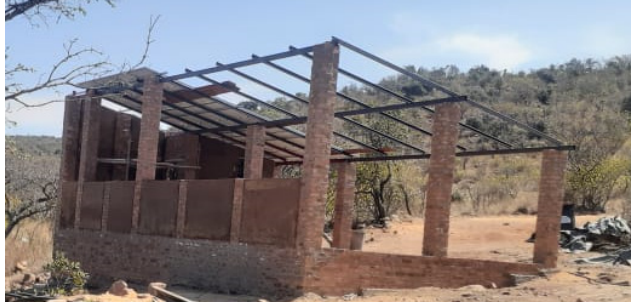
Figure 17: View from south of carport with completed ERE wall panels.
