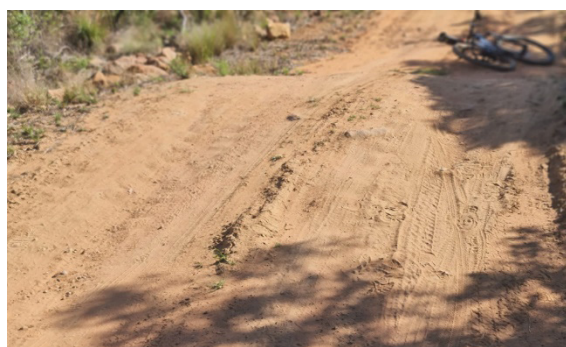
Figure 18: Typical water erosion protection hump.
