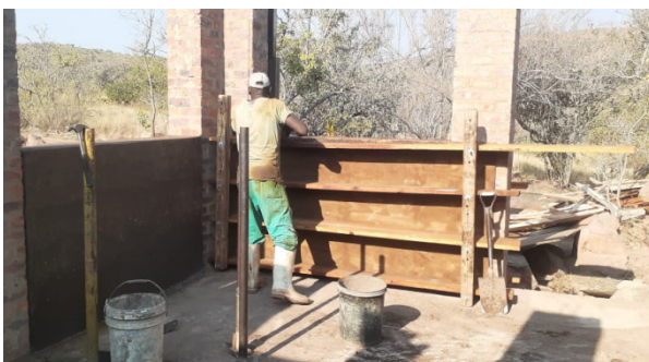
Figure 12: Scaffolding and formwork from inside
