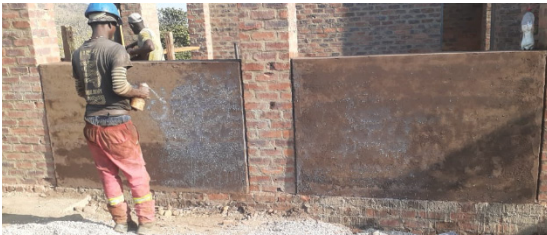
Figure 15. Surface treatment application
