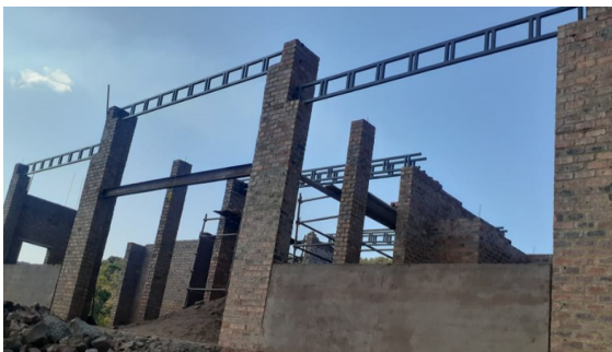
Figure 16. View from the south showing completed low height ERE panels
