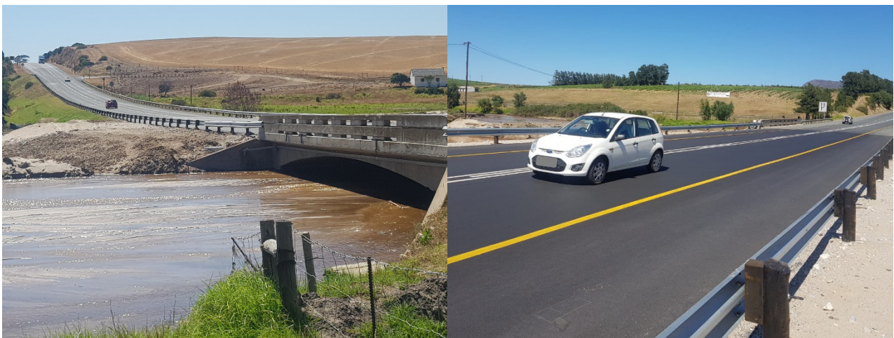
Figure 2: N2 Repair at Bot River (authors own photographs)
