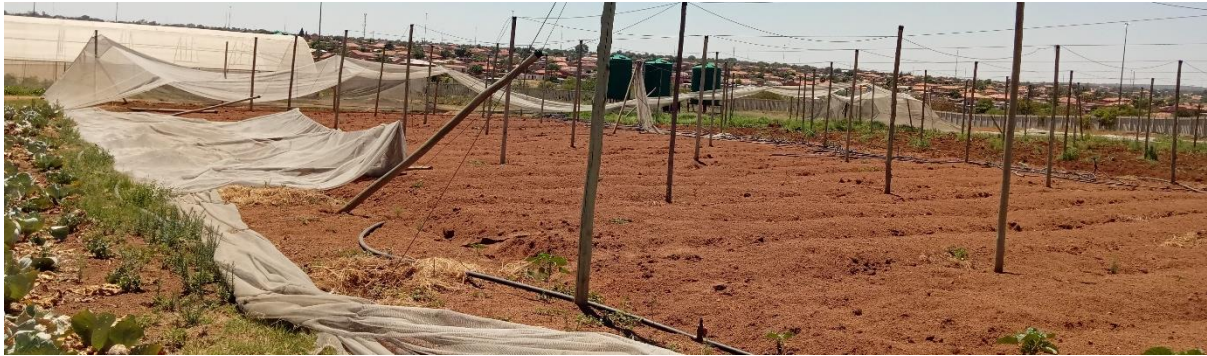
Figure 3-1: Damage at the Soshanguve FPSU test site 2018-12-12
