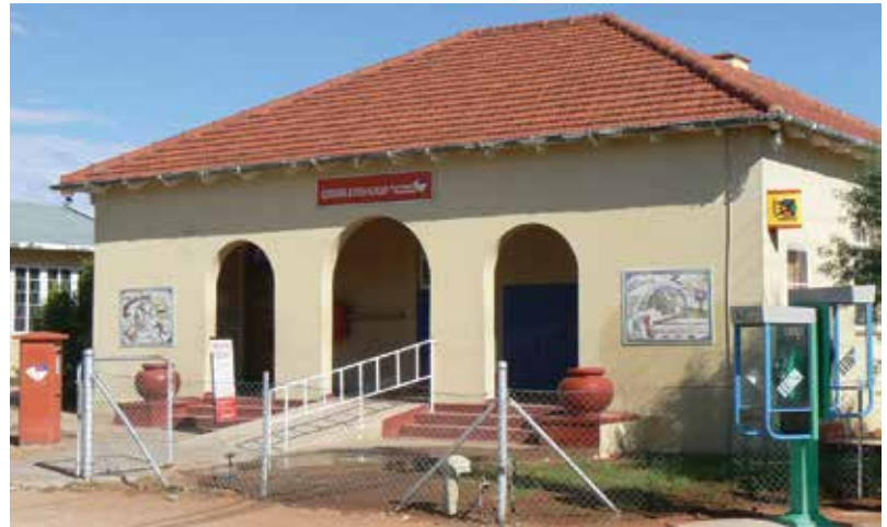
Fig.3: Groblershoop post office indicating the position of the panels.
