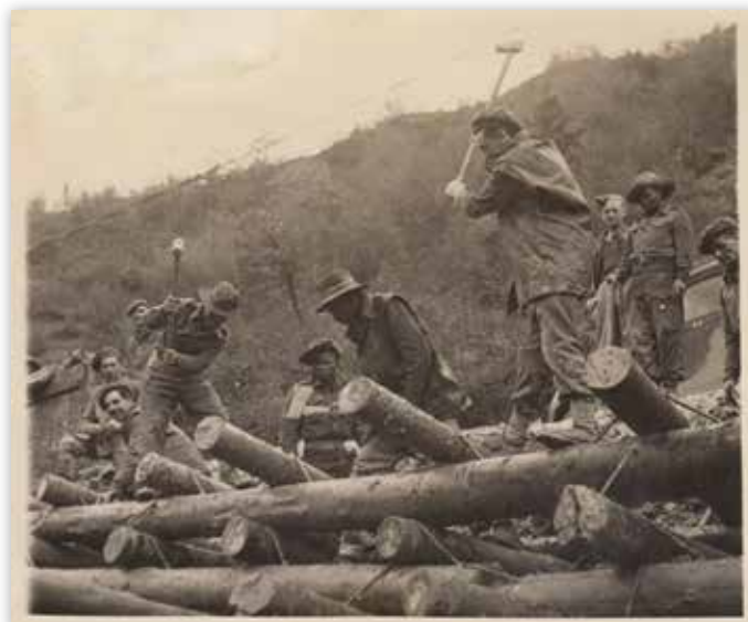
Fig.2: Official Army Field Press photo from 1944 showing a Bechuanaland labour group doing road construction together with Royal Engineers near Castel del Rio, northern Italy.
