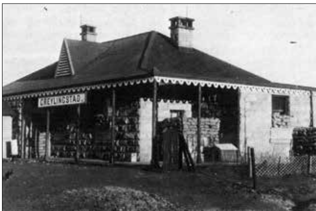
Fig.8: Greylingstad Station converted into a blockhouse by British troops during the ABW by strengthening the outer walls with sandbags. (Source: Todd & Fordham, Private Tucker's Boer War Diary, p. 184).
