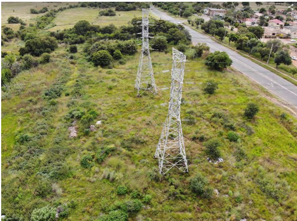
Photo plate 8: Oblique remote image showing the frequent occurrence of Acacia karroo within the Atteridgeville study area
