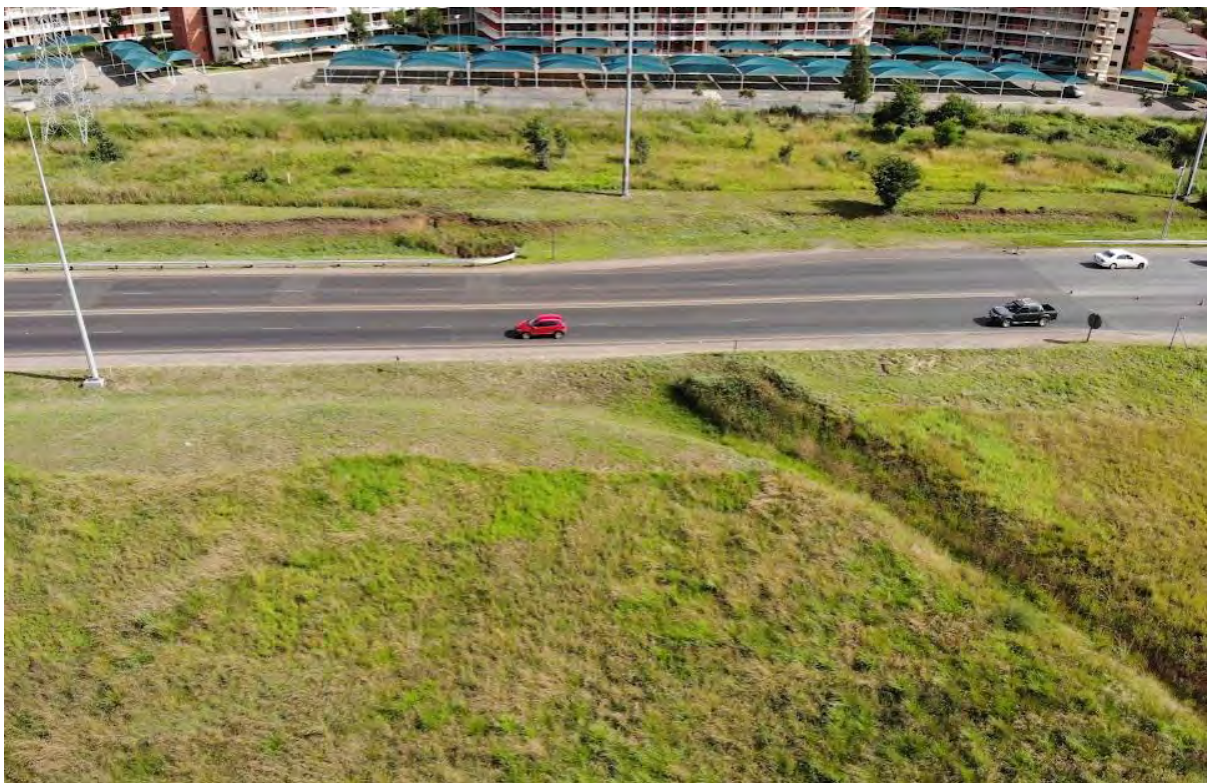
Photo plate 7: Examples of stormwater channels directing excess water to the Atteridgeville study area
