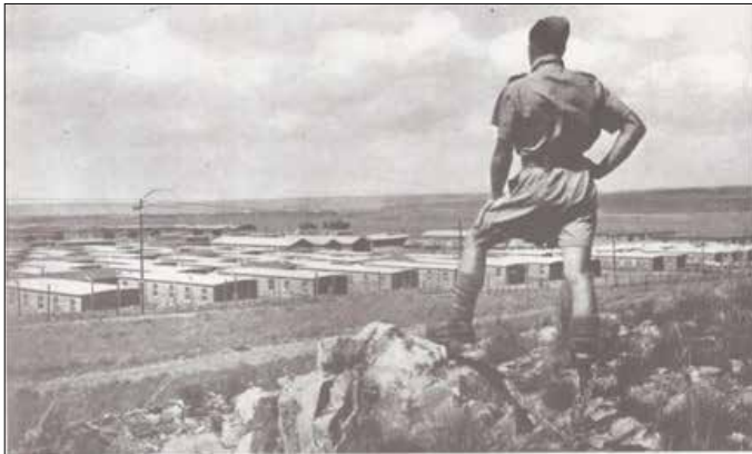
Fig.5: Zonderwater rebuilt as 14 blocks, after completion.
