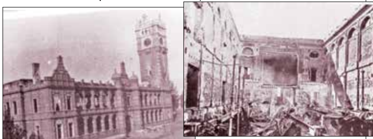
Figs.7 & 8: Photographs of the fire damaged Pietermaritzburg Town Hall (ex Gordon 1981).
