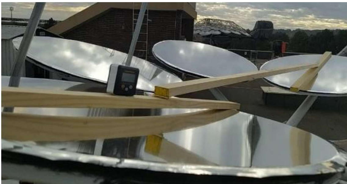
Figure 19. Facet positioning method using a wooden template and digital inclinometer.
