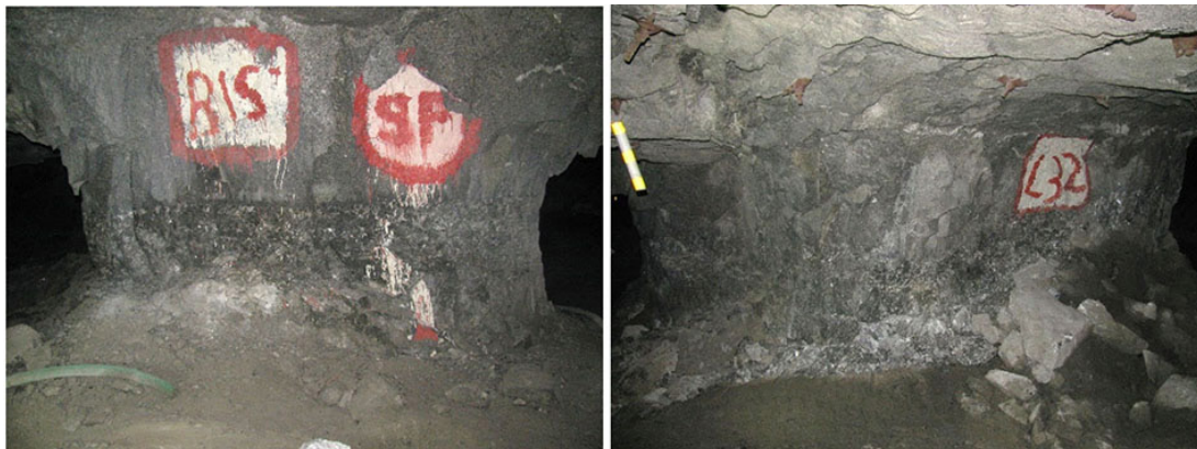
Figure 11—Typical condition of the pillars in the mine selected for the case study
