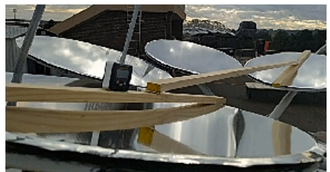
Fig. 3. Facet positioning method using a wooden template and digital inclinometer.
