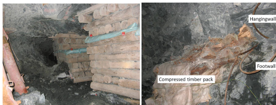
Fig. 1. A deep tabular gold mine stope illustrating typical timber support packs (left). These packs are compressed to a small width if closure occurs (right). (For interpretation of the references to colour in this figure legend, the reader is referred to the Web version of this article.)
