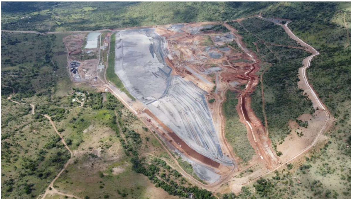
Figure 17 Mareesburg TSF ongoing construction
