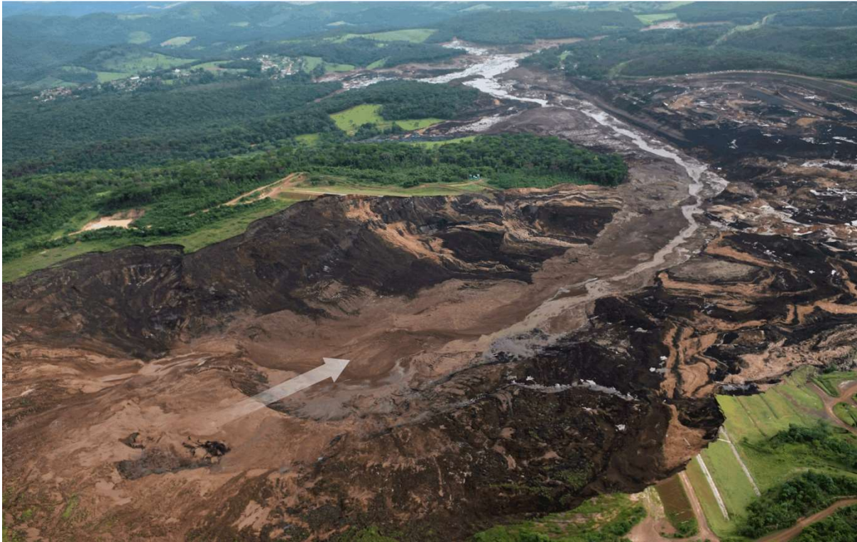
Figure 3 Collapse of the Brumadinho dam in Mina Córrego do Feijo (Piciullo et al., 2022)
