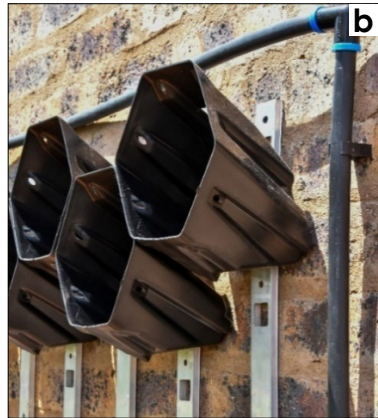
Figure 6b: The pots clip onto aluminium rails, that are fixed to the Future Africa campus kitchen yard wall
