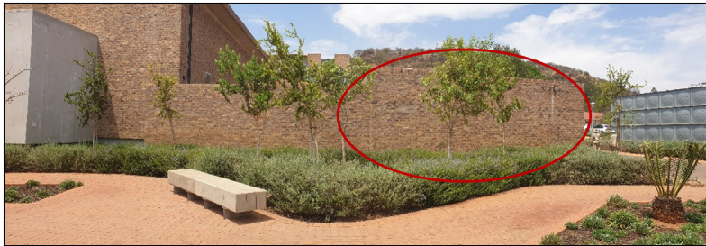
Figure 2: The north-facing kitchen yard wall at the Future Africa campus that was selected as the experimental study site
