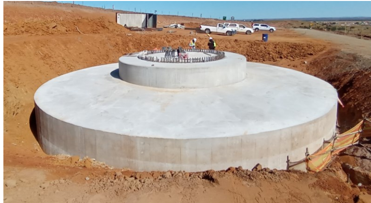
Figure 3-4: Completed WTG09 foundation
