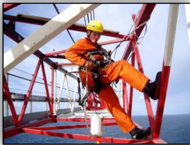
Figure 12- Working above water of unknown depth (e-Architect, 2022).
