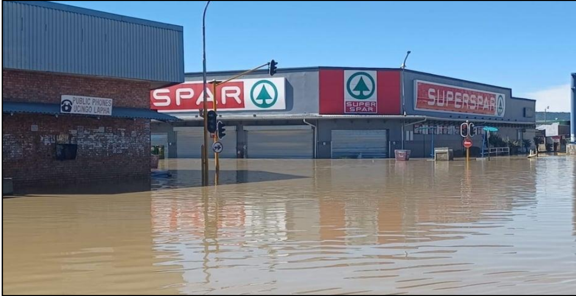
Figure 2-10 Flooding of shops in an area called The Field as a result of floods that hit Durban, KwaZulu-Natal, on 12 April 2022. Source: eNCA, 2023.
