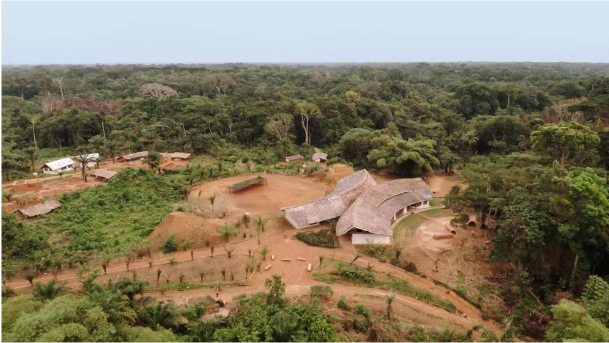
Figure 7.4. Ilima Primary School aerial view (MASS Design Group, 2016)
