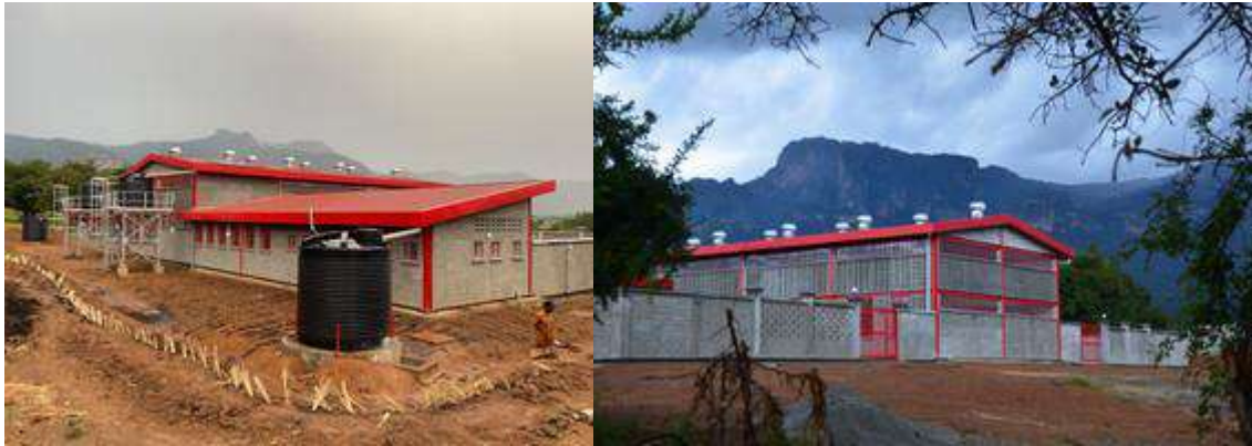
Figure 7.16. Nakapiripirit Vocational Institute buildings (Clegg & Sandeman, 2019)
