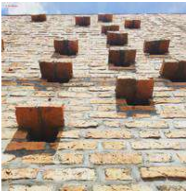
Figure 7.11. Covered perforations on blockwork (Clegg & Sandeman, 2019)
