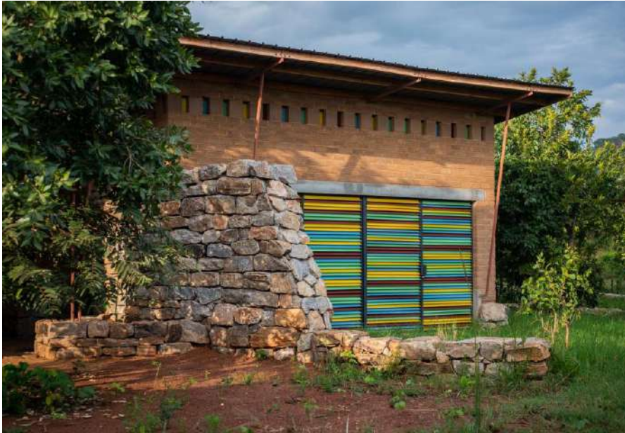
Figure 7.14. Multi coloured louvres (Clegg & Sandeman, 2019)
