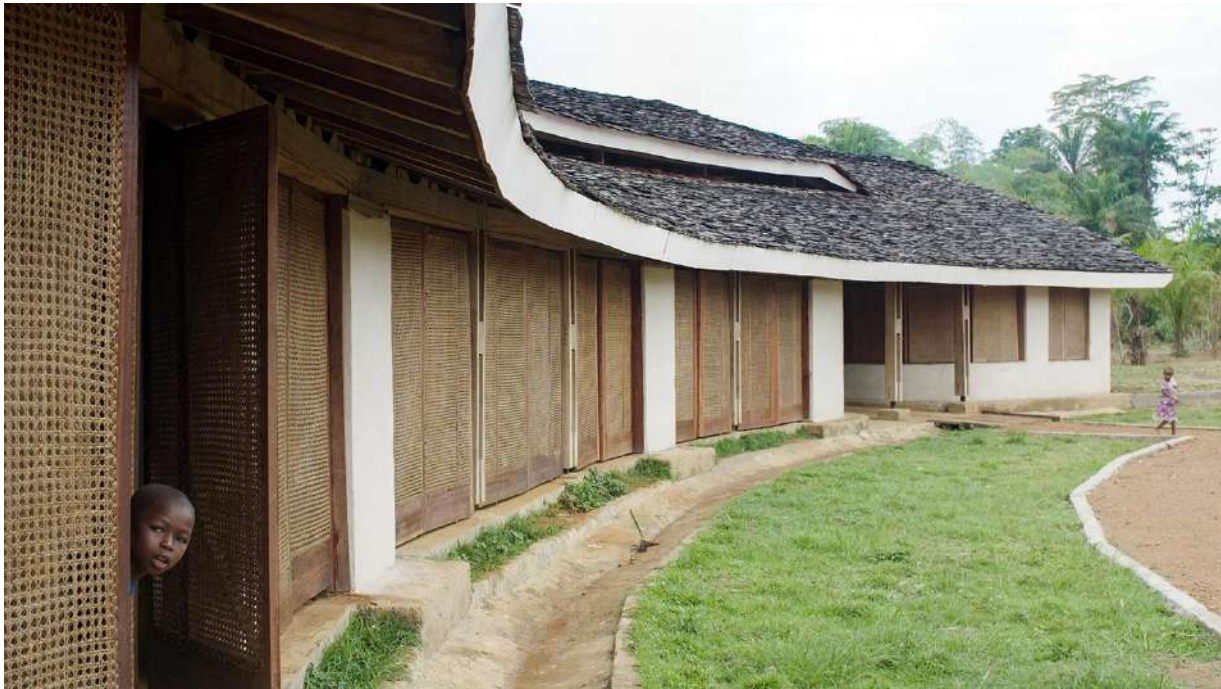
Figure 7.6. Classroom with perforated doors and windows (MASS Design Group, 2016)
