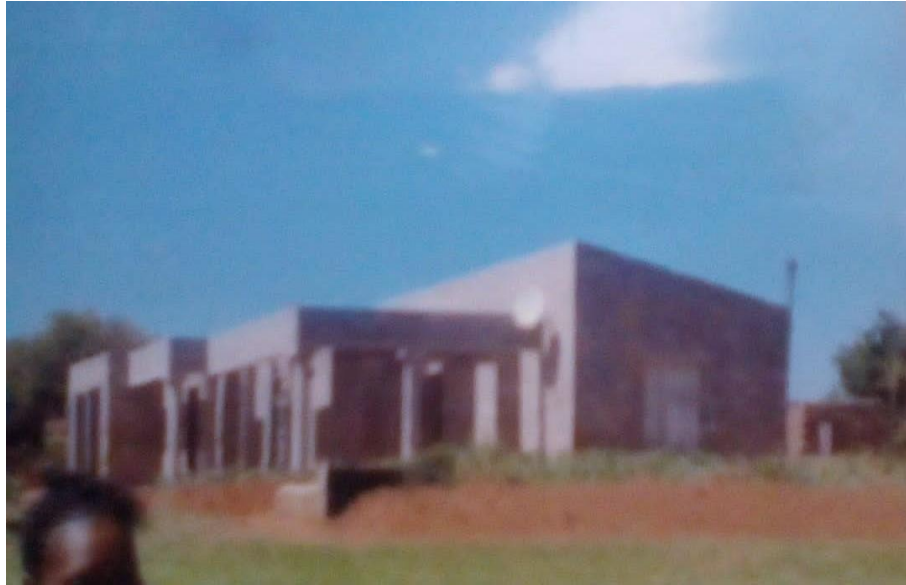
Figure 5.1: Ponts'o's house in the process of extension from two rooms (Source: Ponts'o's archives)
