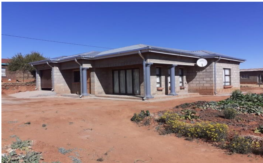
Figure 5.2: Ponts'o's house after extension and renovation (Source: Author, 2021)
