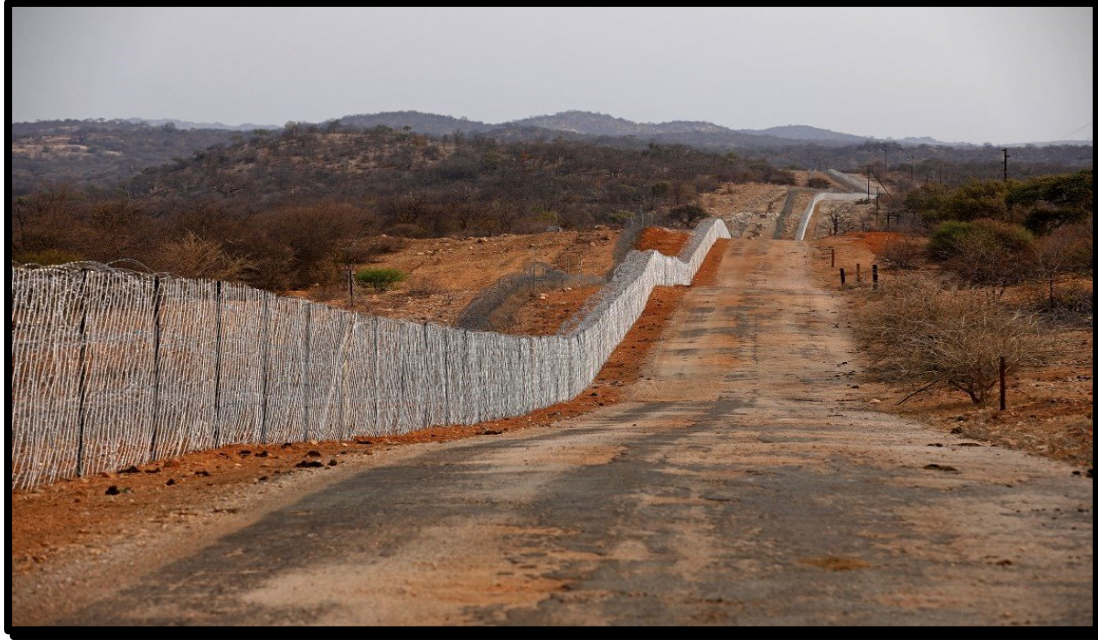
Figure 4.5: The new fence that was completed in April 2020
