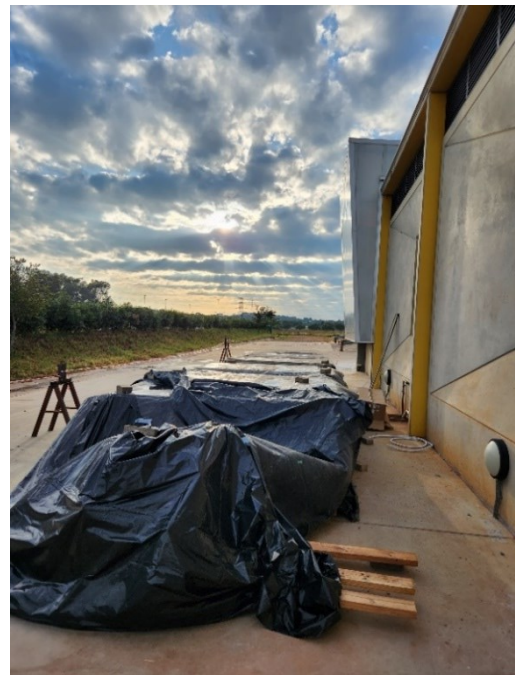
Figure 3-19 Curing blankets placed over beams
