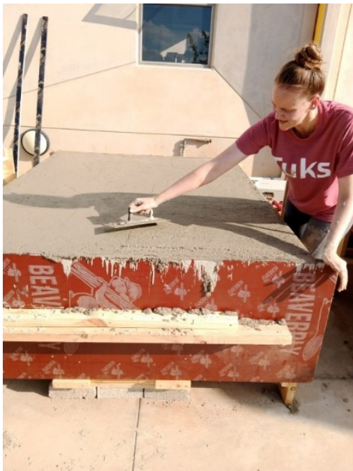
Figure 3-18 Concrete surface floating
