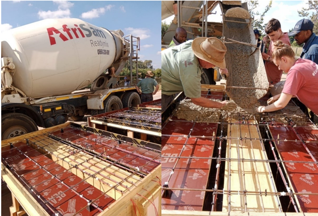
Figure 3-17 Moulds and concrete mixer truck before and during casting
