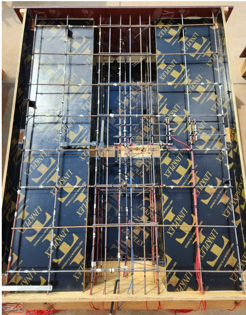
Figure 3-7 Solid T-beam mould with reinforcement cage
