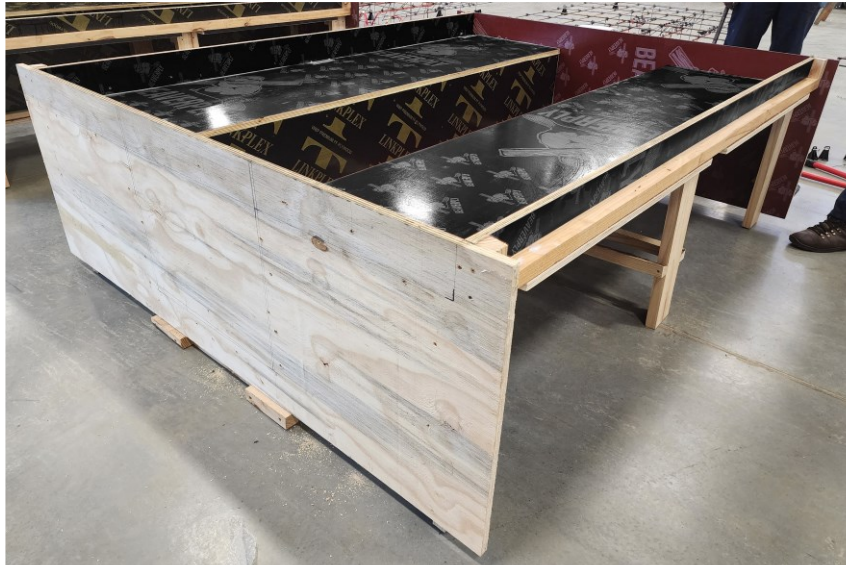
Figure 3-6 Completed solid T-beam mould
