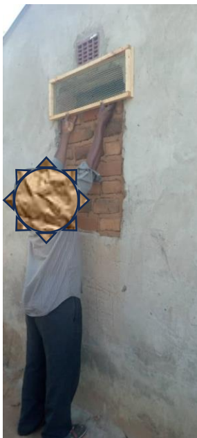
Figure 3a: Placing the GNT over a ventilation space in a room used for sleeping.
