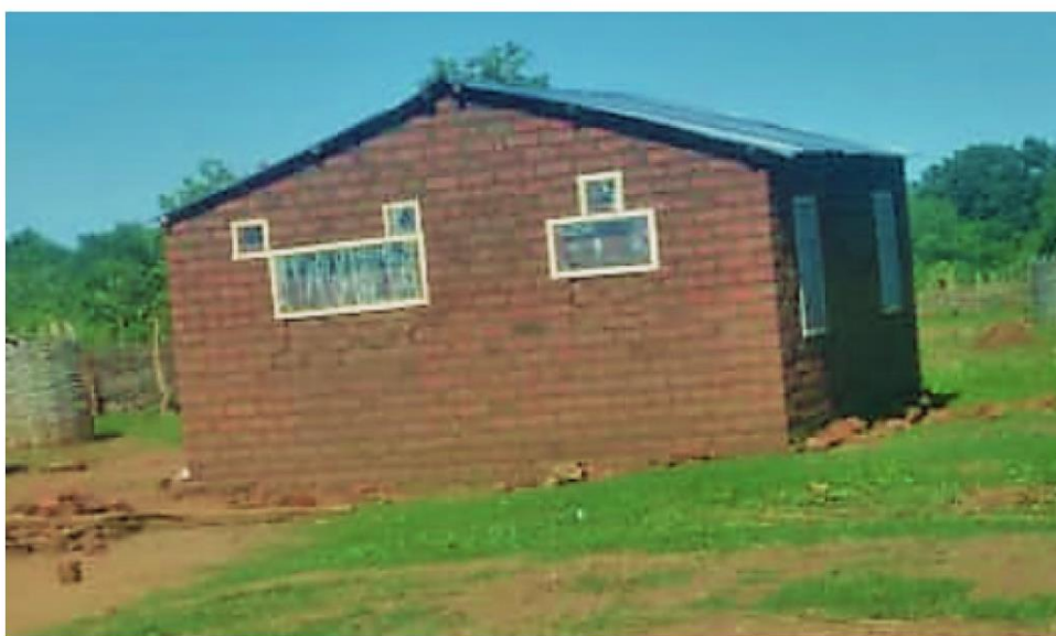
Figure 2. A semi-modern house with firebrick walls and a metal roof showing screened windows and ventilation spaces.
