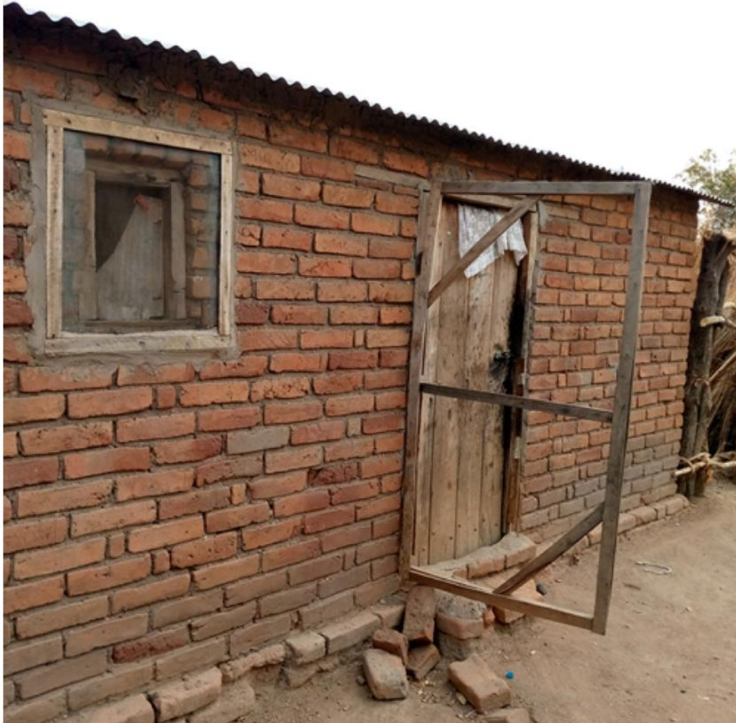
Fig. 4 Completely removed wire gauze on a door screen frame
