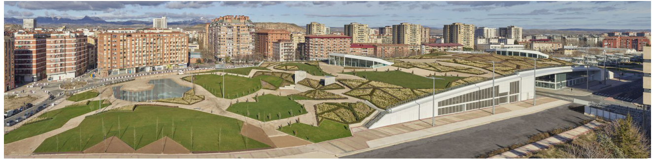
Figure 11: Aerial view of the Logrono station (Archdaily 2023)
