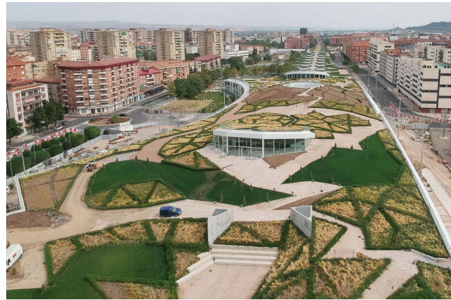
Figure 12: Aerial view of the Logrono station (Archdaily 2023)
