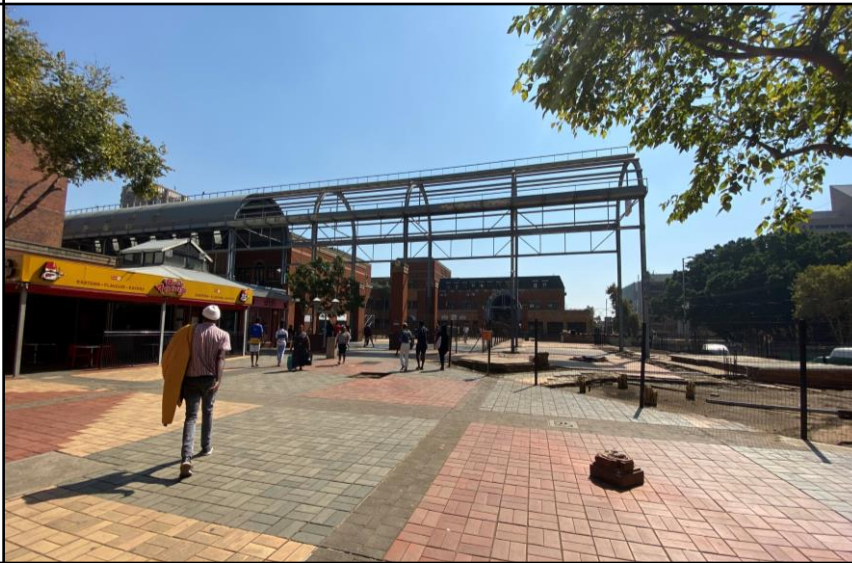
Figure 3: Existing Sammy Marks Square, South East Entrance
