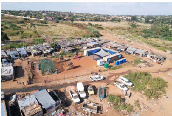
Figure 3: SA Cares for Life creche school aerial photo 2)
