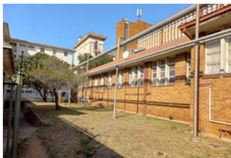
Site photos from East
