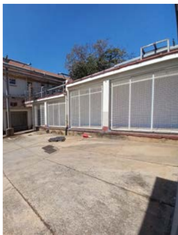
Covered walkway blocking axis
