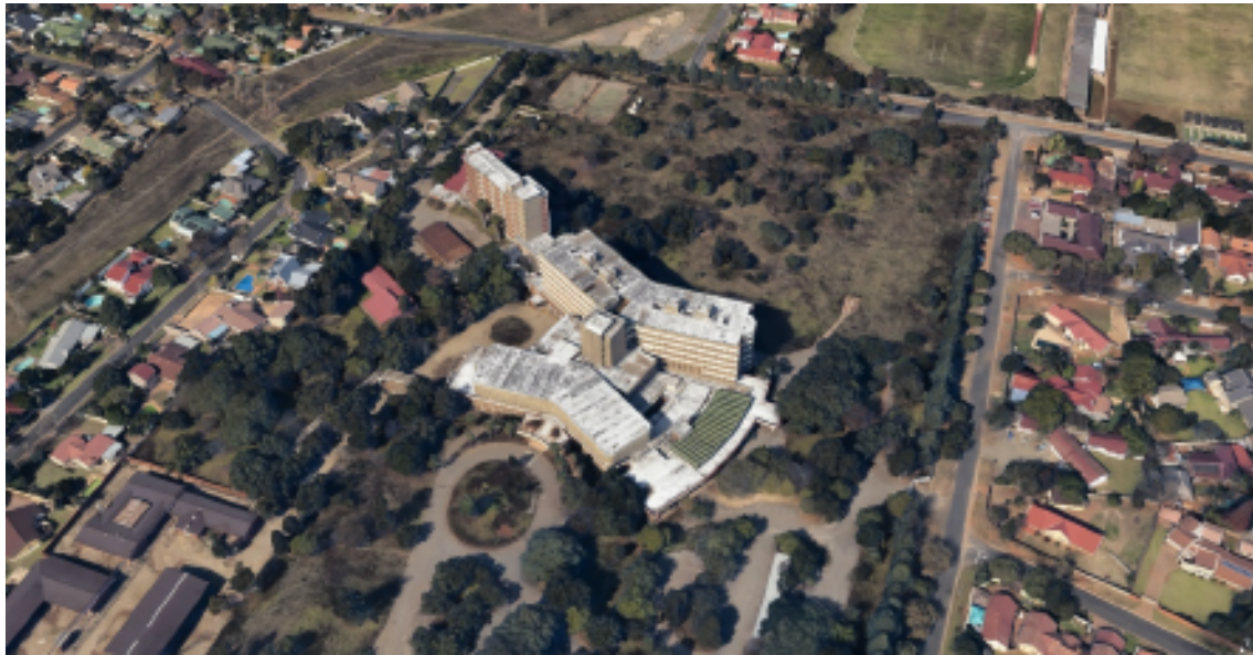
Figure 109 Kempton Park Hospital (abandoned) (Google,2023)
