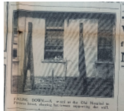
Figure 77 Volkshospitaal wall damage (NARSSA, 2023)
