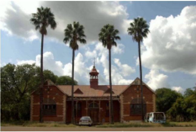
Figure 58 Westfort administration building (Clark, 2016)
