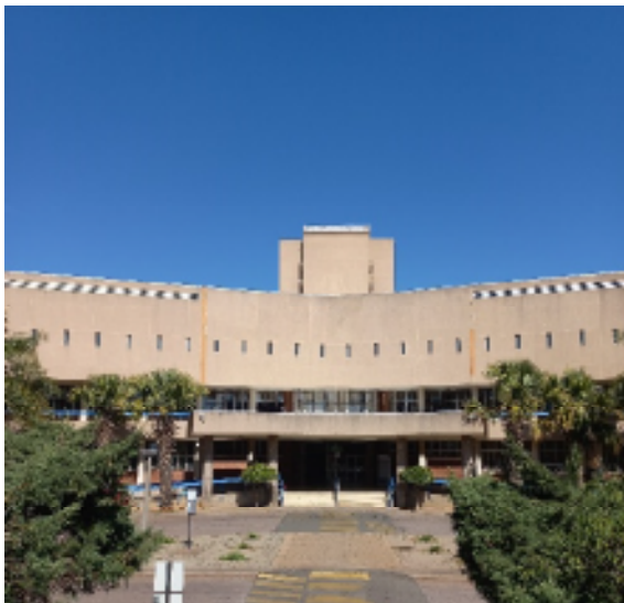
Figure 34 Pretoria west hospital (author)
