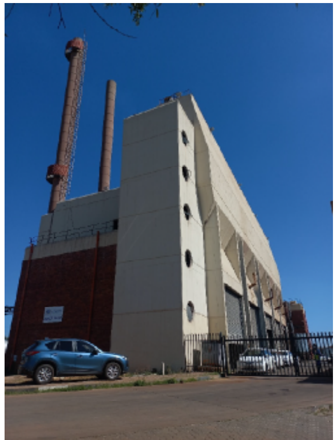
Figure 119 Dr George Mukhari Hospital Boiler room (author)
