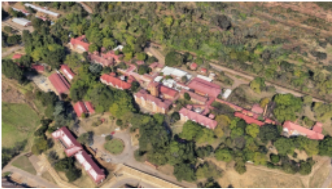
Figure 38 Weskoppies hospital (Google, 2023)
