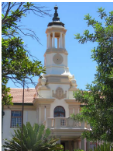
Figure 72 Tshwane District administration building (Fisher, 2023)
