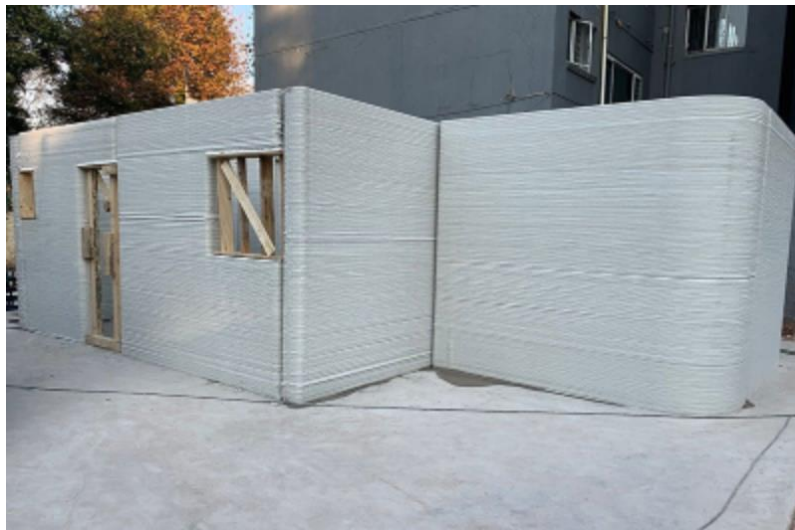
Figure 21 - South Africa's first 3D printed low-cost house by University of Johannesburg's civil engineering department (2022) - Project 17 (Reporters at News24, 2023)
