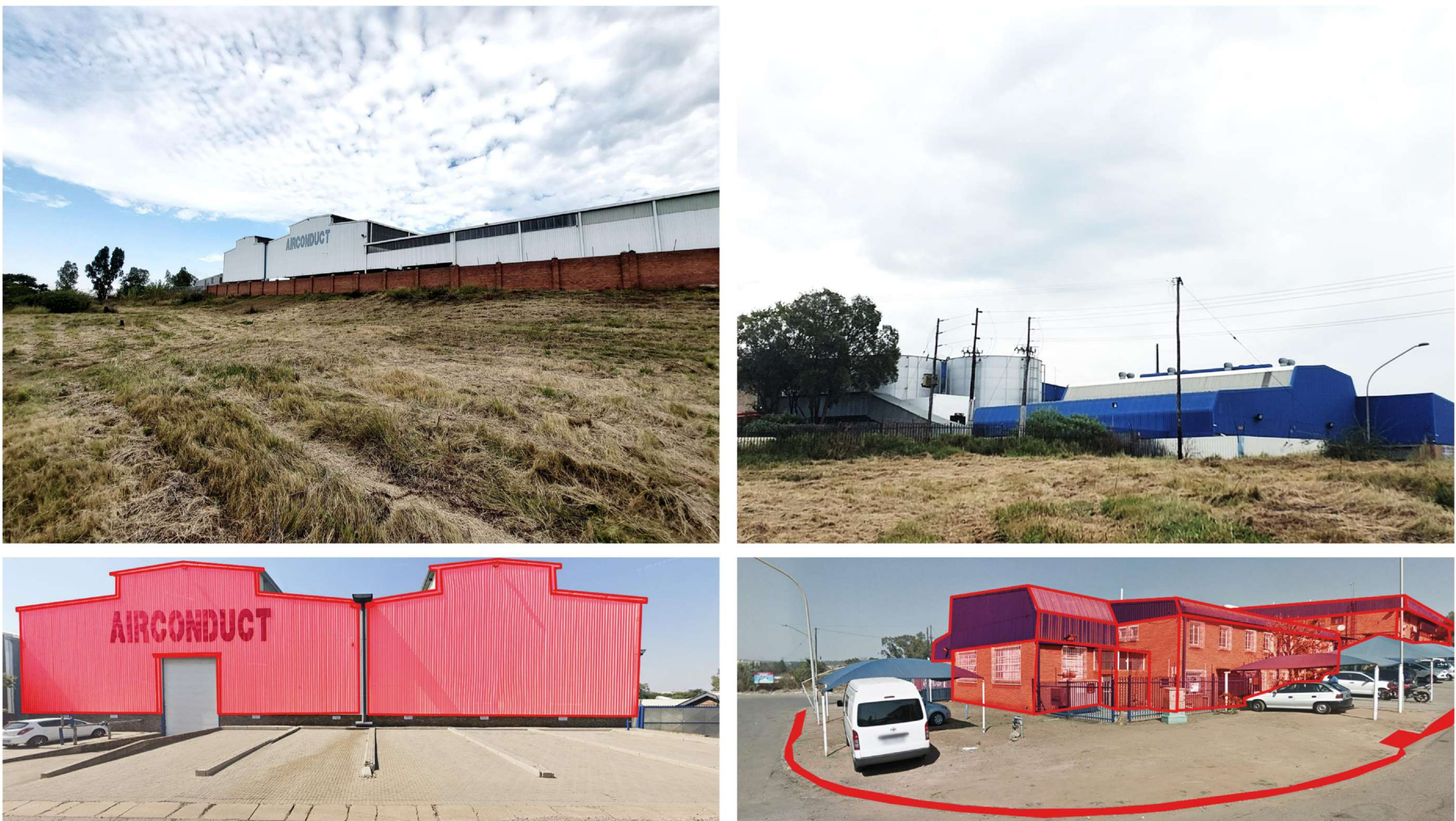
Figure 4: Adapted pictures taken on site visit (Author, 2023)
