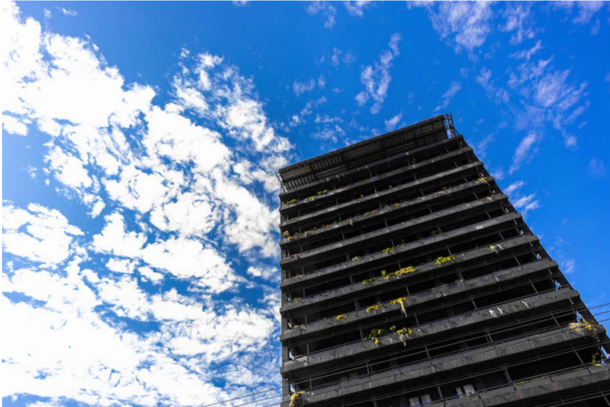
Figure 15: The 66-metre high Modernist structure of Hallmark House, initially designed in the early 1970s as a diamond-polishing factory and later repurposed and designed by distinguished Ghanaian architect David Adjaye (Hallmark House n.d.).
