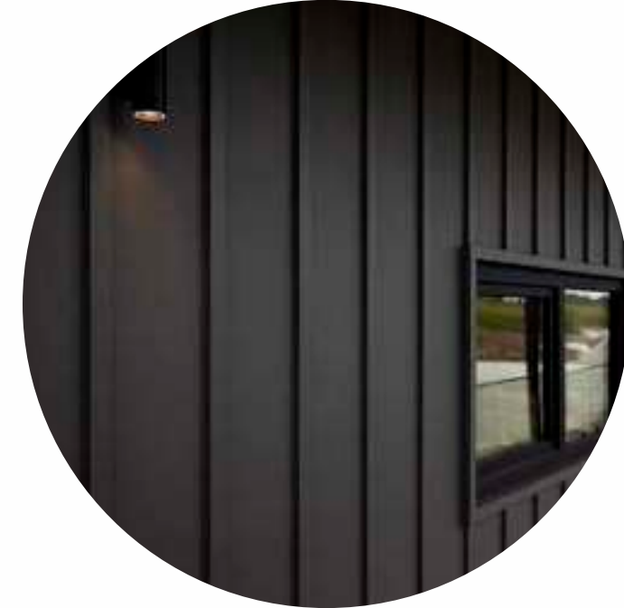
Vertical fibre-cement interlocking shiplap boards (image by James Hardie)
