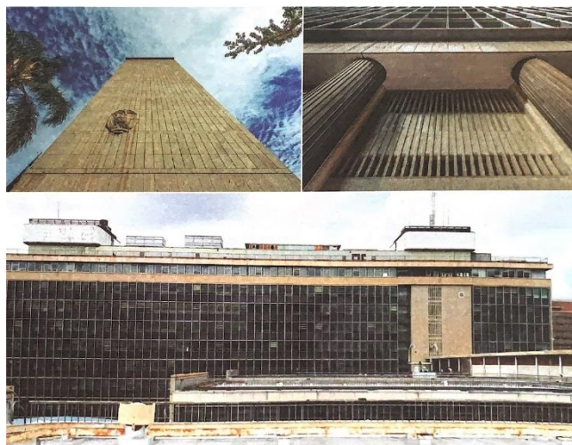
Figure 9: The abandoned TPA Building on Church Square (Swart, 2023).
