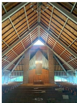
Figure 36: Interior with A-frame steel structure and timber lattice work (Author, 2023).
