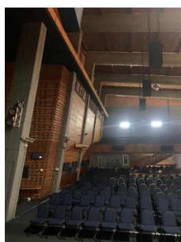
Figure 62: The structure of the building remains intact (Author, 2023).
