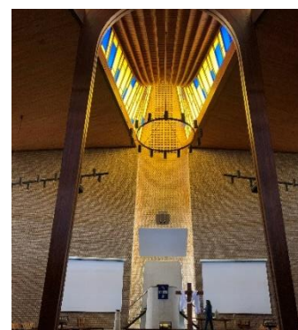
Figure 57: Laminated timber trusses and clerestory windows above the pulpit (Author, 2023).
