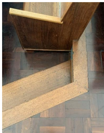
Figure 25: Original materiality still in good condition (Author, 2023).
