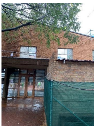
Figure 53: Construction of student housing on the site (Author, 2023).
