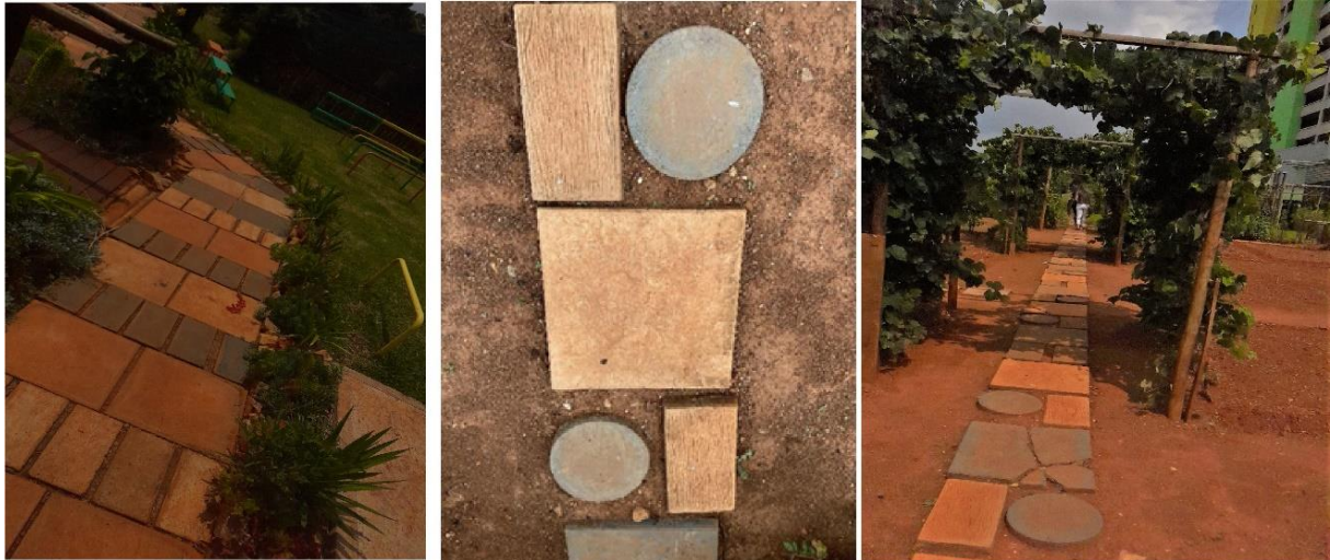
Figure 7: Different types of Stone Paver paths in the site. Some accessible [left] Some inaccessible [centre and right] (Author, 2023).
