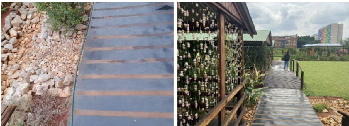
Figure 6: Textured Rubber and Timber walkway along the North Boundary Cabins. (Author, and Mnguni ,2023).
