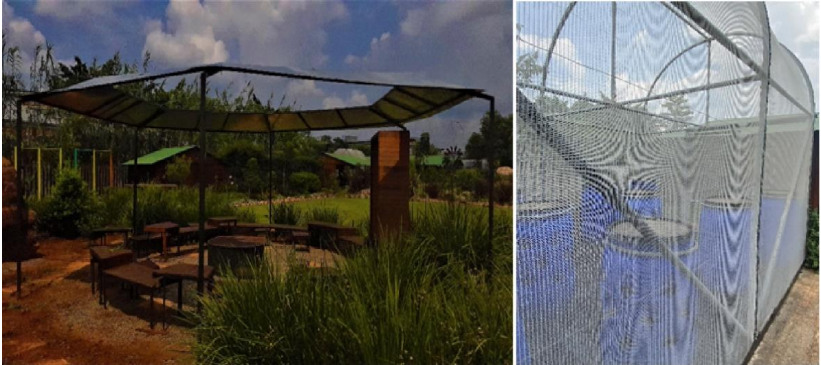
Figure 5: Steel structures on site- Left: Gazebo; Right: Hydroponic greenhouse (Author, du Plessis, 2023).
