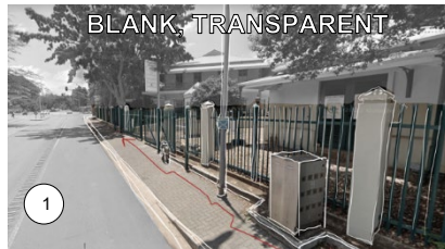
Figure 52: Obstructed sidewalk along Arcadia Street (Author, 2023).
