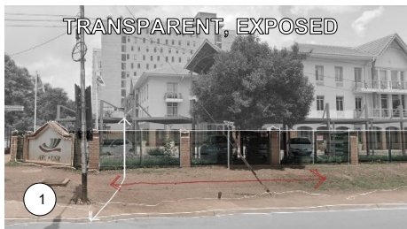
Figure 45: Uncomfortable sidewalk conditions (uneven and exposed to traffic) with lack of shading framed by a blank, transparent interface along Grosvenor Street (Author, 2023).
