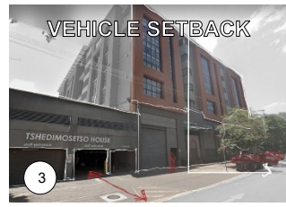
Figure 41: Vehicle setback interface obstructing pedestrian movement (Author, 2023)
