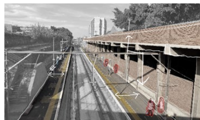
Figure 71: Lack of seating and shade for commuters of the Metrorail (Author:2023)
