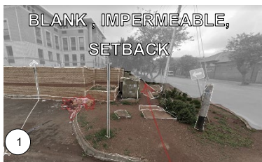
Figure 39: Dumping and sidewalk obstructions along framed by a blank interface (Author, 2023).
