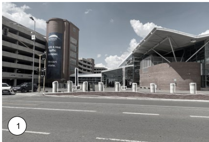
Figure 73: A lack of activity surrounding the Gautrain station (Author:2023)
