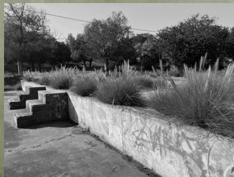
Fig. 9. Site Photo: Uncompleted infrastructure, left as concrete islands in the landscape.
