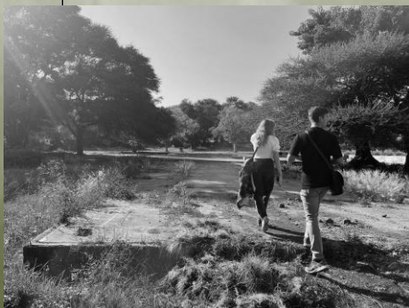
Fig. 7. Site Photo: Foundations and infrastructure not completed and left to decay. Nature taking over the redundant former infrastructure.
