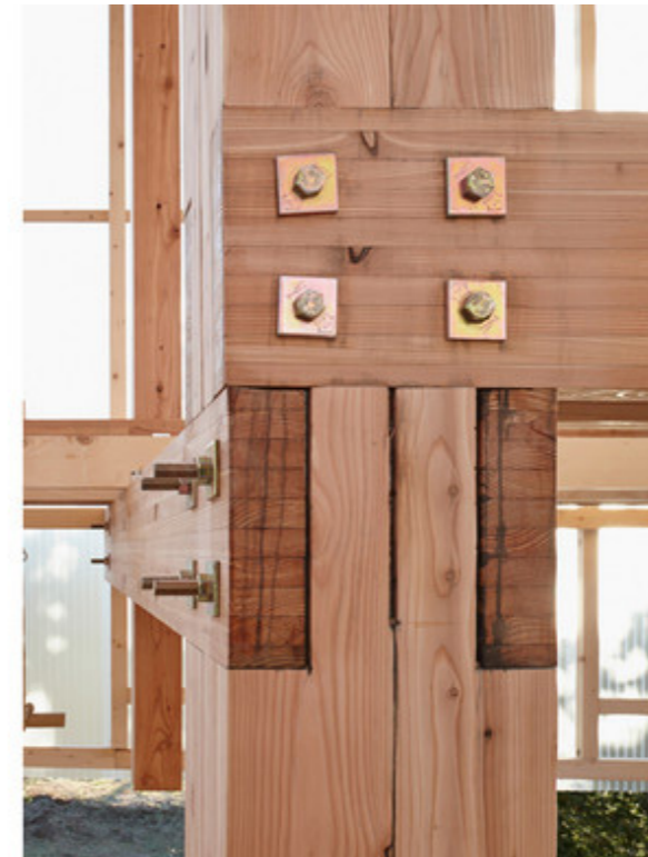
Figure 2: Timber detailed column connection ("Nest we grow" by Kengo Kuma)
