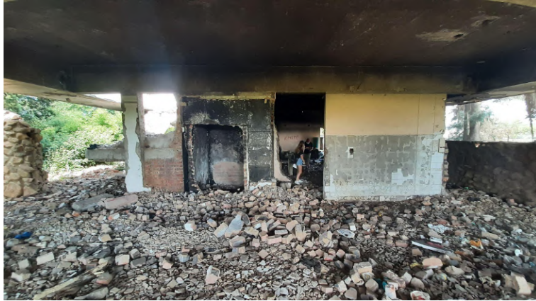
Figure 3.15 - Derelict Beerhall in Atteridgeville, with broken bricks that can be upcycled into non-load bearing walls (infill walls), pathways, gabion structures, landscaping and foundation infill (Author 2022).
