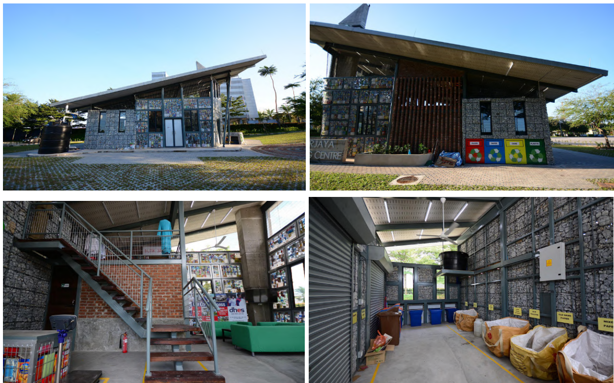
Figure 2.5 - Cyberjaya Recycling Centre showing recycling (Top) and rock (Bottom) infill walls in steel frame. (ATSA 2017)
