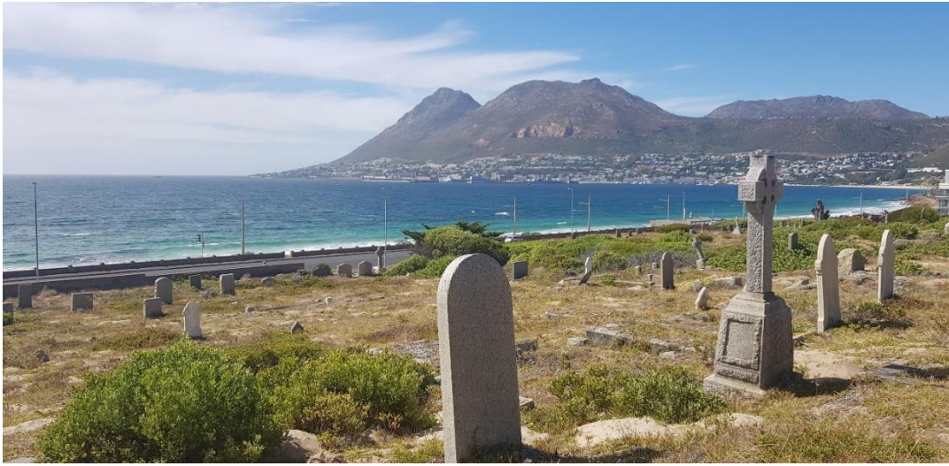
Figure 11. Tombstones in Dido Valley Cemetery, Simon's Town. Note in particular the lack of tree cover and proximity to the ocean, suggesting that these tombstones are likely to be constantly exposed to salt-laden wind
