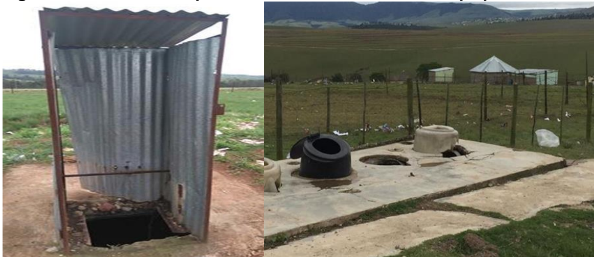
Figure 5.20: Evidence of pit latrine toilets in the Eastern Cape province
