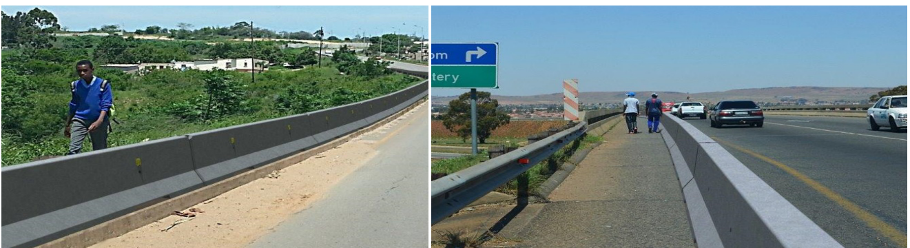
Figure 2: Examples of correct crash tested and installed VRS that offer protection to VRUs
