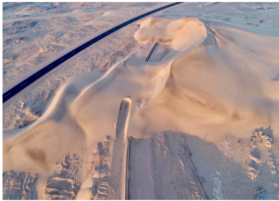
Figure 1: Aus- Lüderitz railway line covered by windblown sand crossing the line
