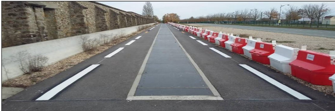
Figure 5: The Satory Test Track right after installation on December 2nd 2019
