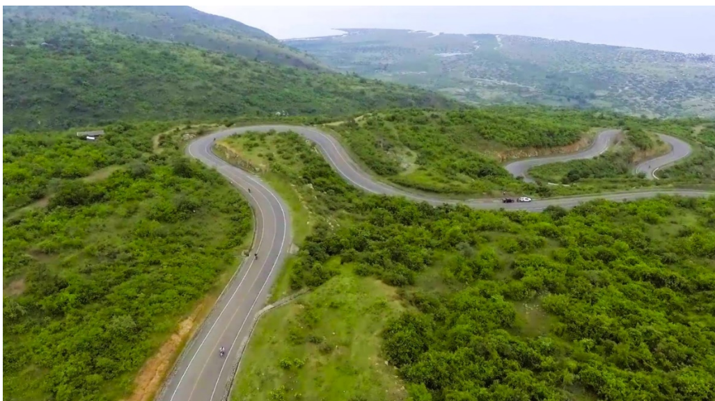
Figure 2: The road to Buliisa district after construction (Photo credit: The Petroleum Authority of Uganda)
