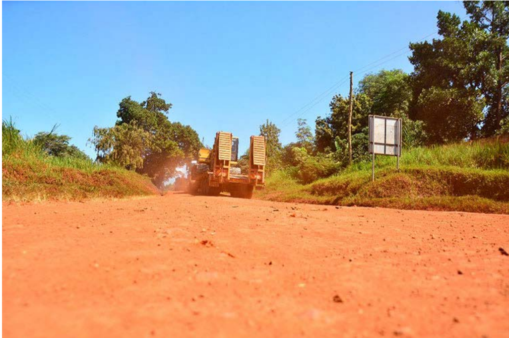
Figure 1: One of the roads under construction (Photo credit: The observer publication)
