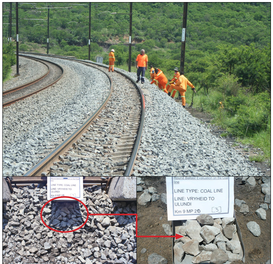
Figure 2 Position of ballast sampling below the sleeper
