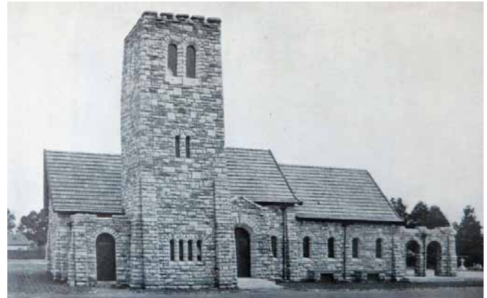
Figure 21: Braamfontein Crematorium in the Year of Its Completion, North Elevation, (1930), Johannesburg Heritage Association.
