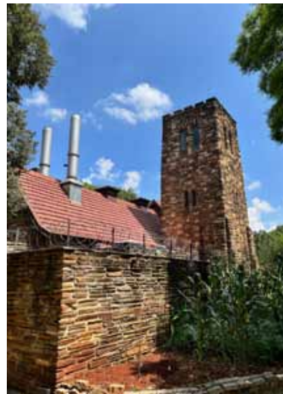
Figure 4: Braamfontein Crematorium with Steel Chimney Stacks, 2022
