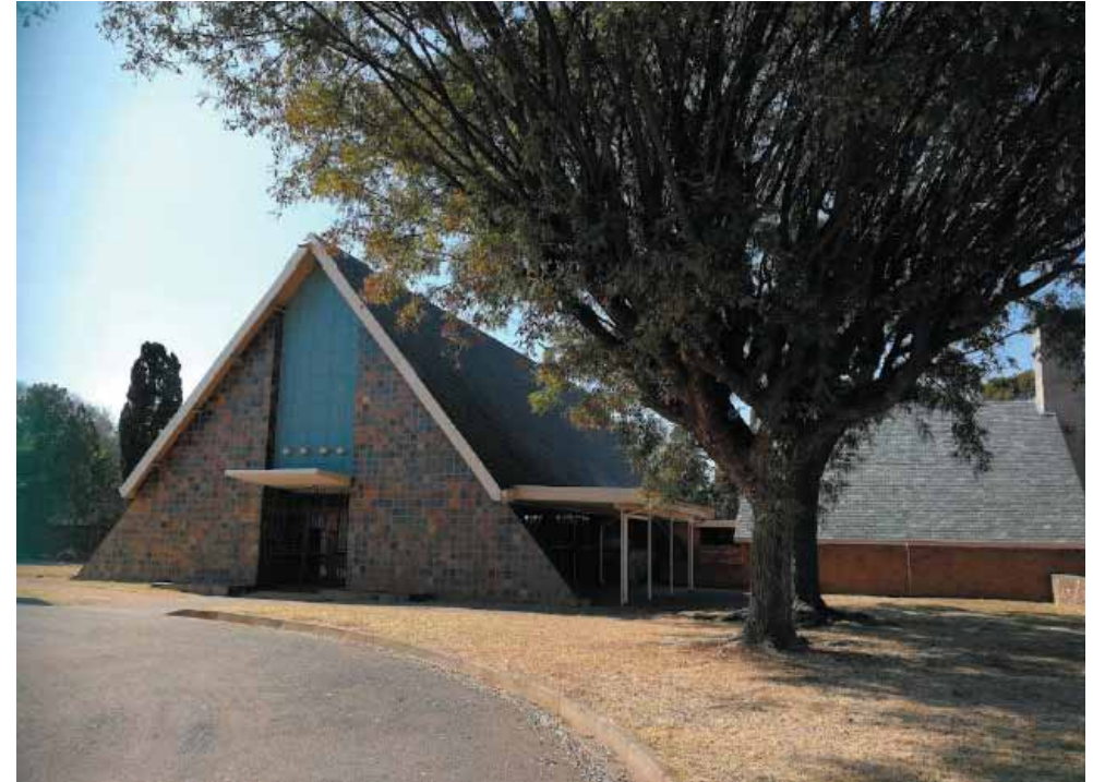
Figure 26: The Rebecca Street Crematorium, Pretoria, Constructed in the mid 1960's, [online]
