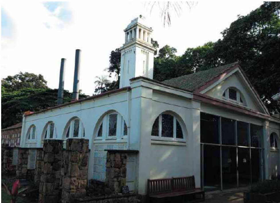
Figure 25: Stella-Wood Crematorium, Durban, Constructed in 1939, Architect: Unknown [online]
