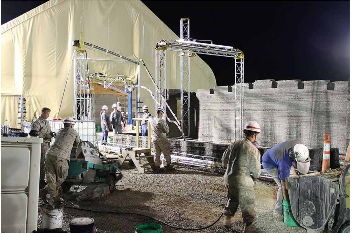
World's largest concrete 3D printer
