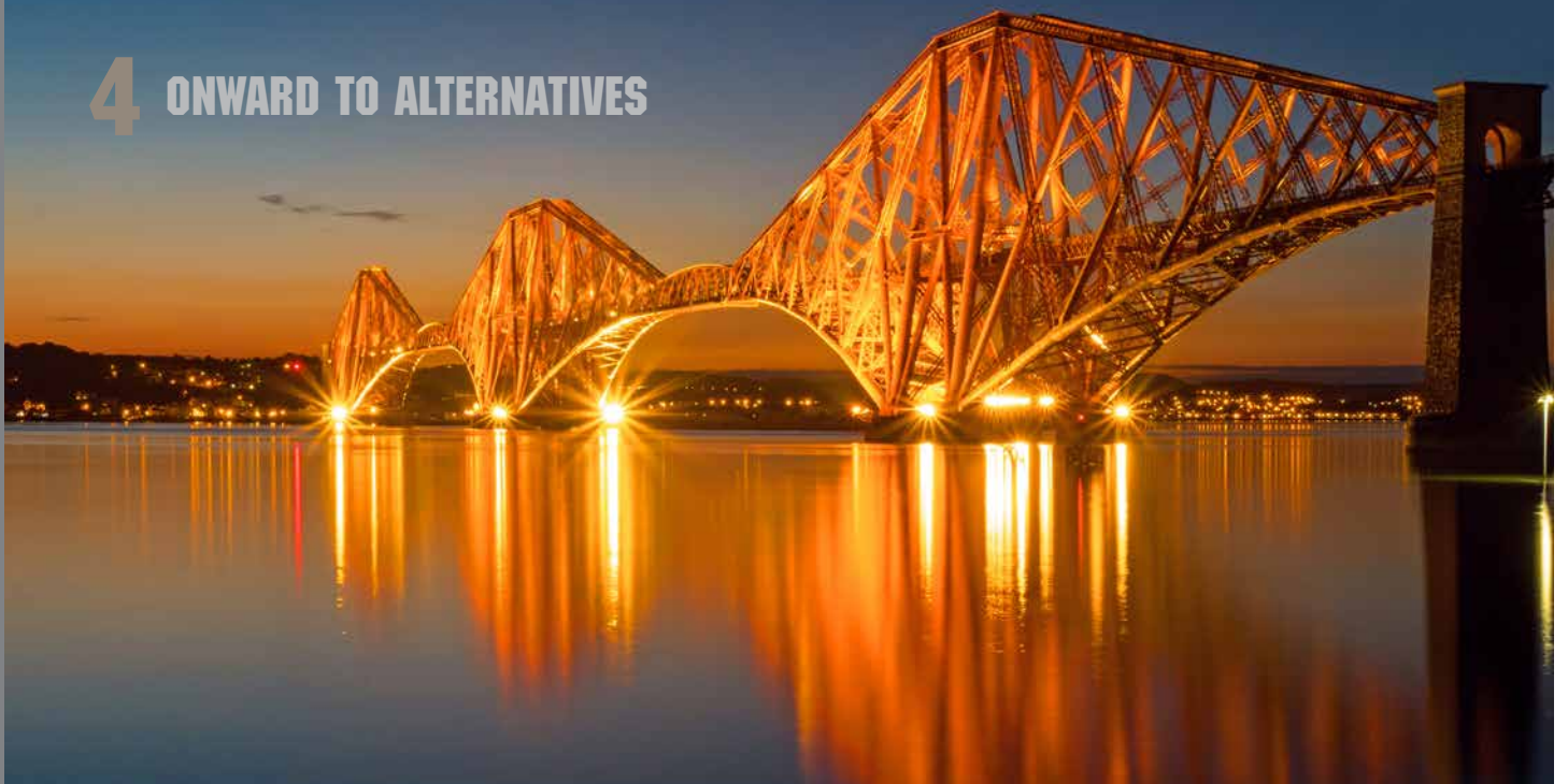
Figure 7: The Fourth Rail Bridge – 8 years to build (1890)
