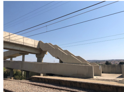
Figure 38: Existing pedestrian bridge crossing the railway (Author)
