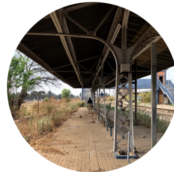
Figure 129: Steel construction (Author)
