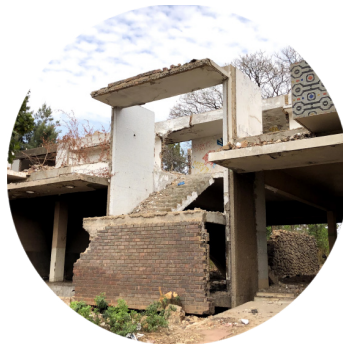
Figure 131: Concrete, brick and mosaic (Author)
