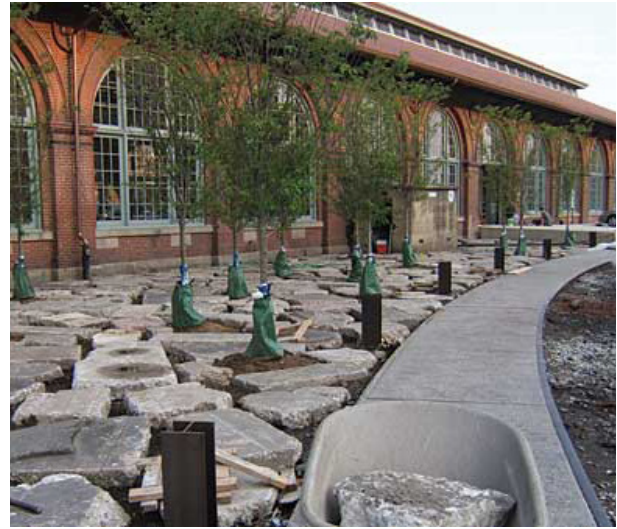
Figure 89: Ordering of salvaged concrete on site (Margolis 2007)
