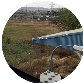
Figure 128: Steel construction (Author)
