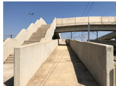
Figure 39: Existing pedestrian bridge crossing the railway (Author)
