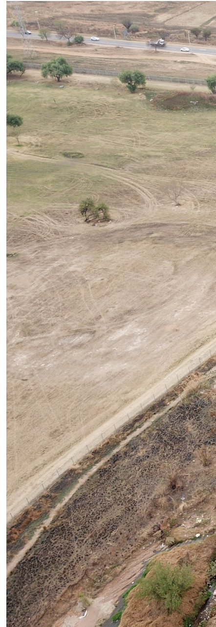
Figure 66: Aerial view of area for technification (Kusel
