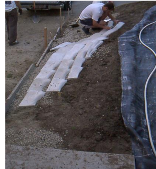
Fig 164: Pre-casted concrete system Being installed on site (Cortex 2004).
