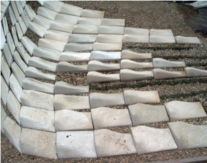
Fig 162: Pre-casted concrete system almost done installed (Cortex 2004).
