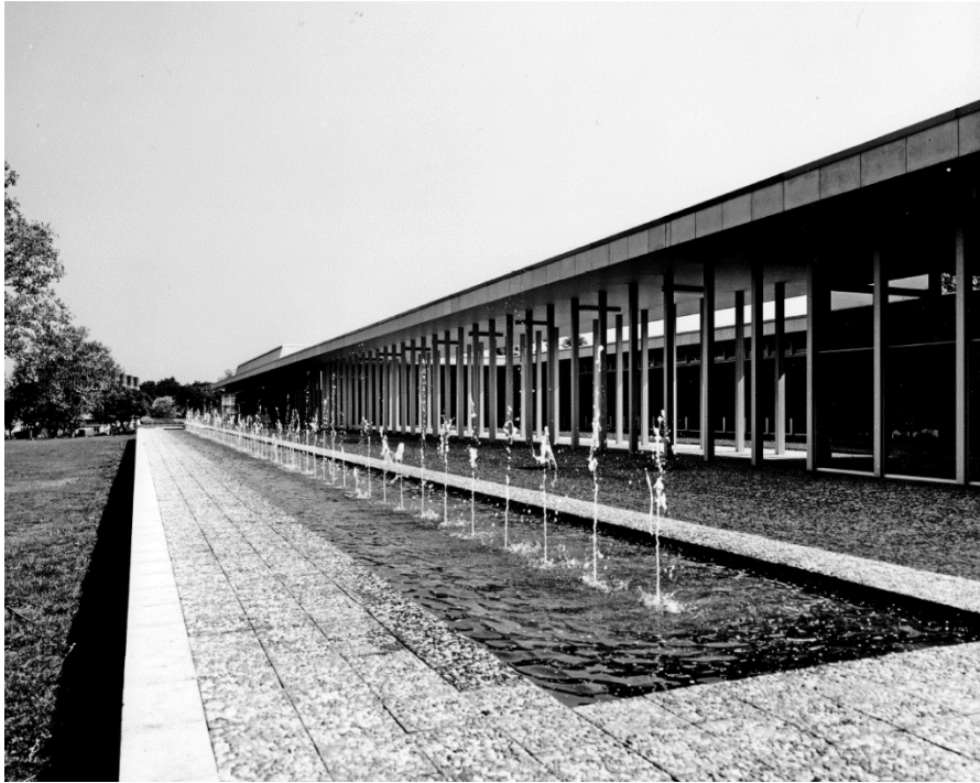
Fig 35: Previous sculpture garden courtyard behind colonnade (Lodge & Burg 1963).
