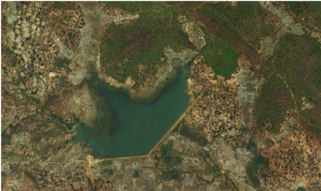
Fig. 2. Satellite view of the reservoir location
