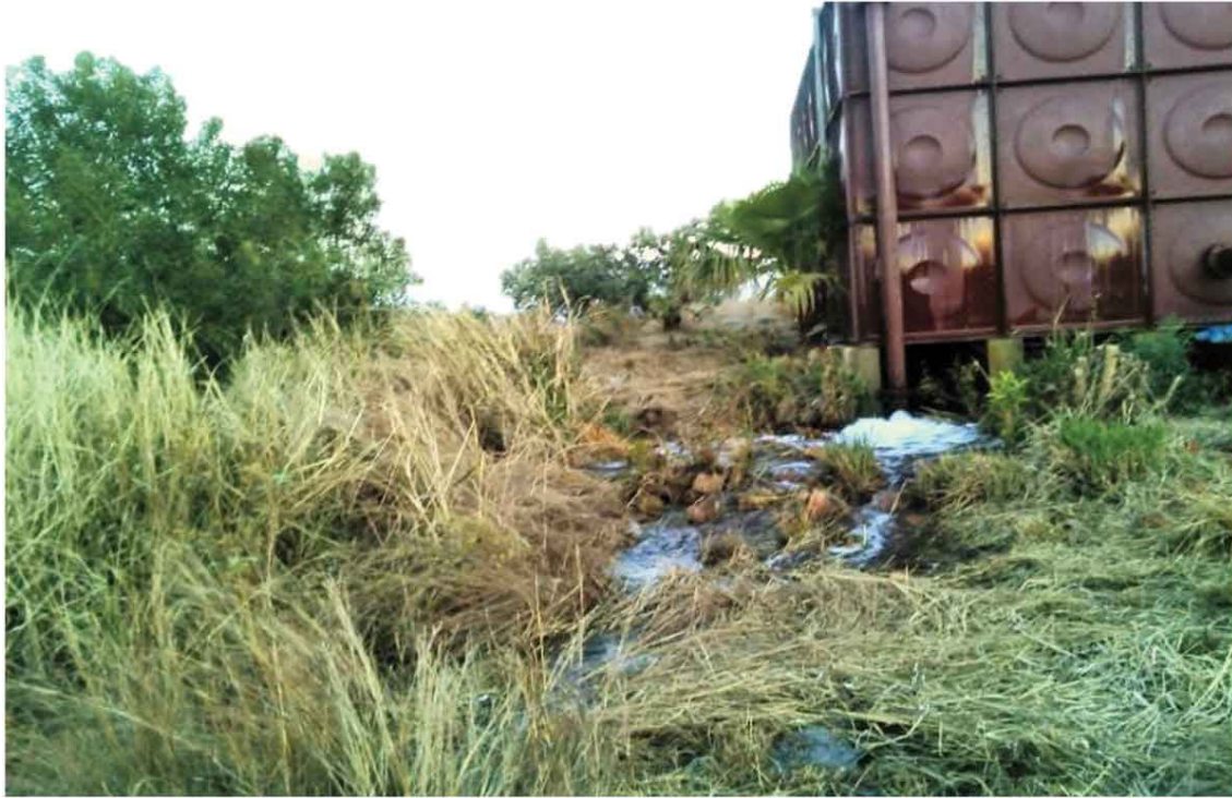
FIGURE 4. The water pump and storage infrastructure leak adjacent to the Kgaswane Mountain Reserve, taken on 9 August 2018
